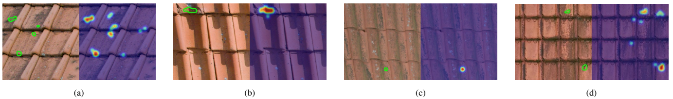
Fig. 15: Incorrect Prediction for Defective Tiled Roof - Right image depicts heatmap of potential defects on the resized original image, while the left image shows the contour overlay of the heatmap for precise localization of defects - The model could not detect defects in a, c and d. In b the defect is too small.
