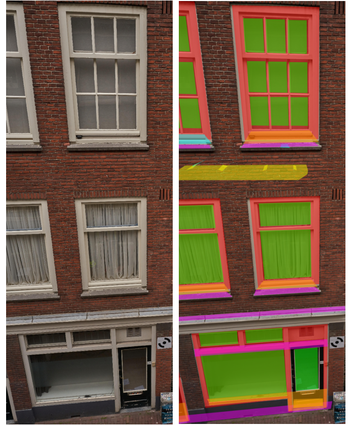
Fig. 2: An image and masks of the casing components and defects on it. Masks for casings, glasses and different defects overlaid onto the original images
